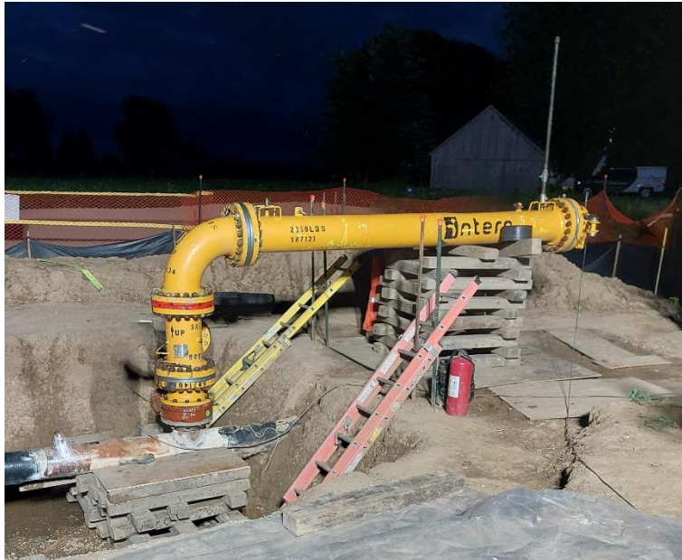
Figure 5. NPS 12 launch and receive site with Interro temporary launcher | Rural site
