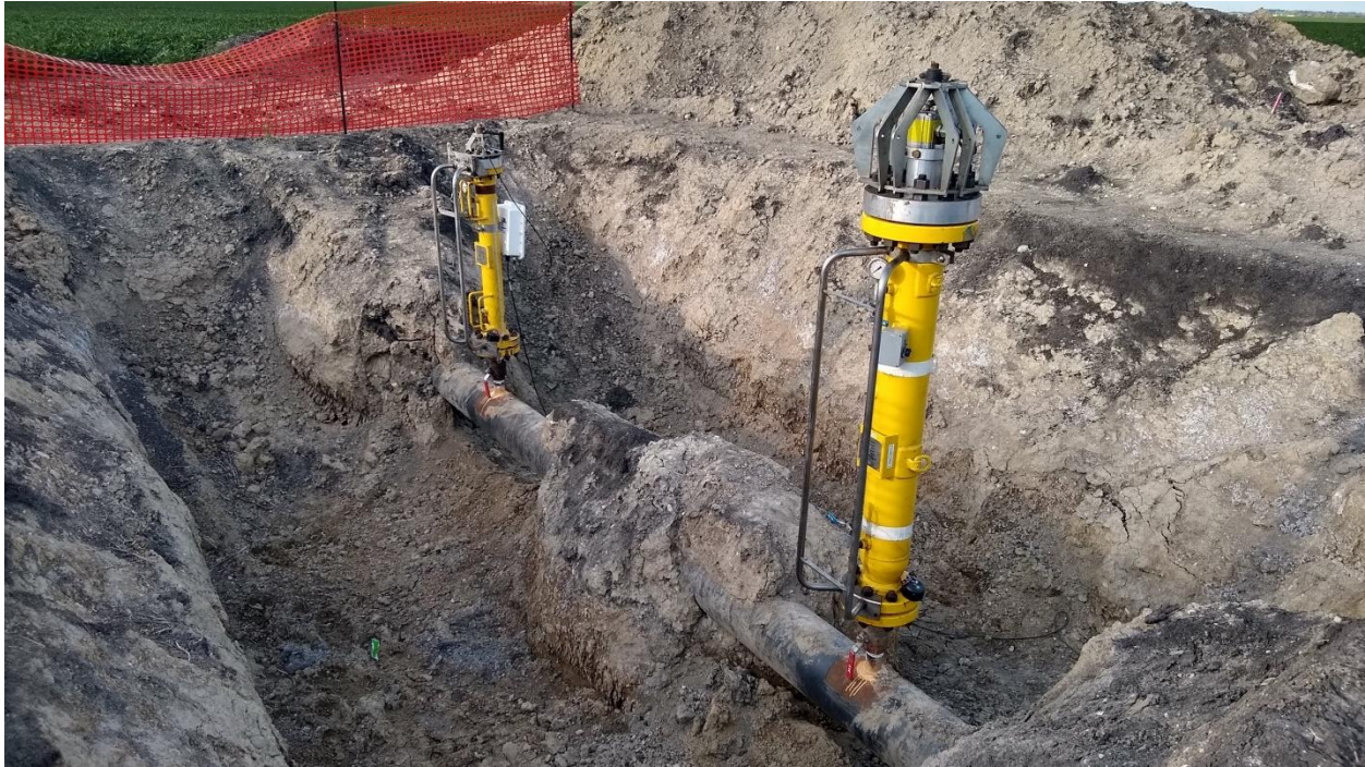
Figure 5: In-line Charging Site on 10 inch Pipeline
