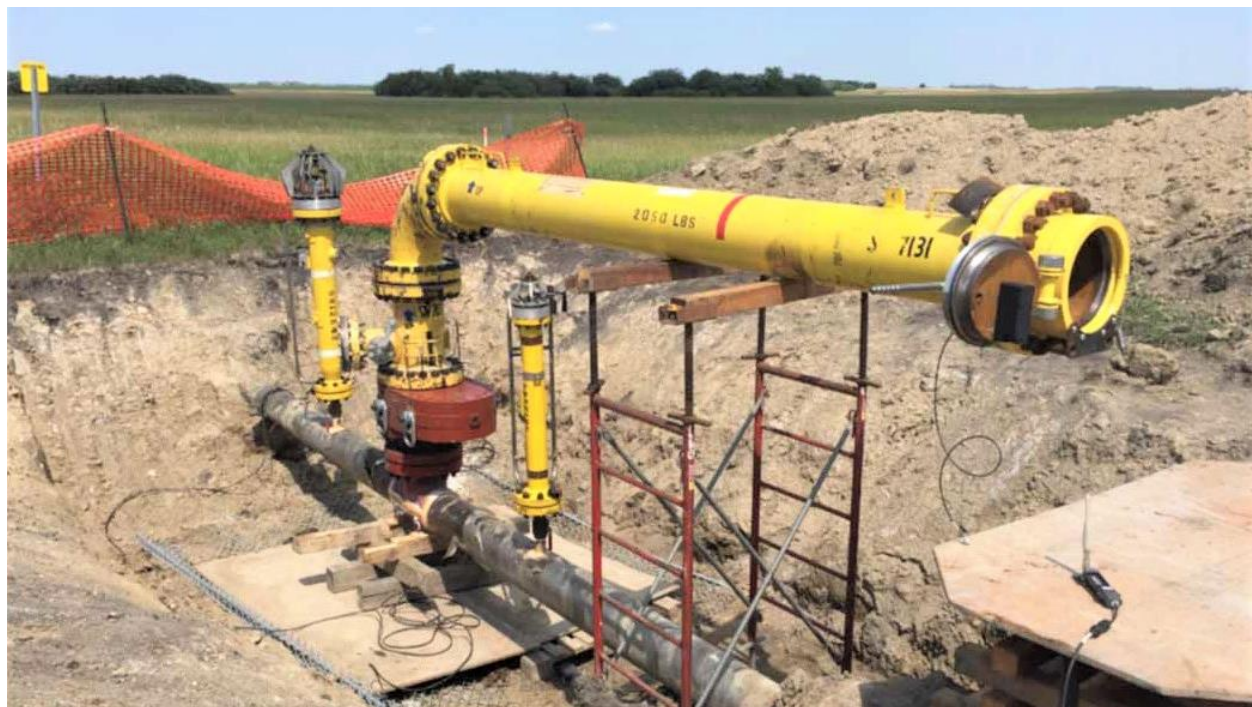
Figure 6: Intero's Launch System for Pipe Explorer 10/14
