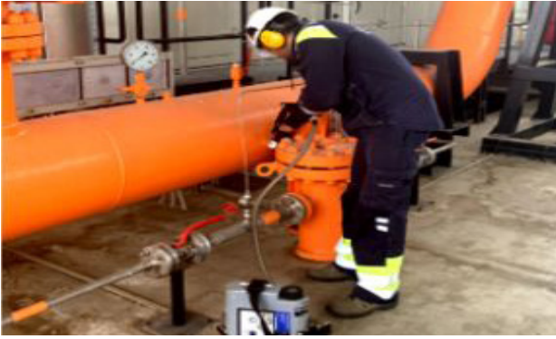
Detecting fugitive methane emissions with an FID / PID measurement device.
