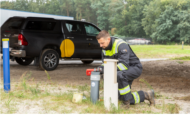
Cathodic protection survey
