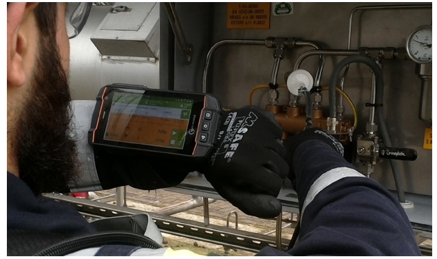
Leak Detection And Repair with the SFEMP Mobile application to collect emission data.
