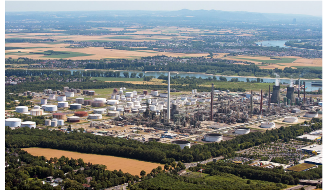
Shell Rheinland refinery in Godorf
